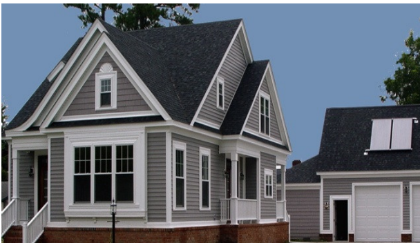
New Home in Raleigh, NC, with SolarH 2 Ot Collectors. Courtesy of SolarH 2 Ot
