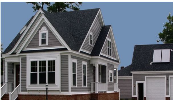
New Home with SolarH 2 Ot Collectors. Courtesy of SolarH 2 Ot
